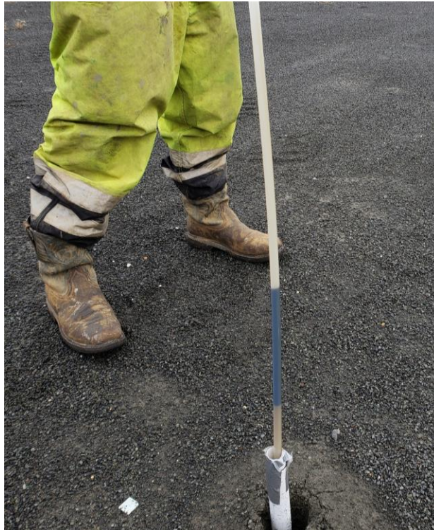
View of approximately one-foot of product measured within TWP-22 (Boring FPA-22).
